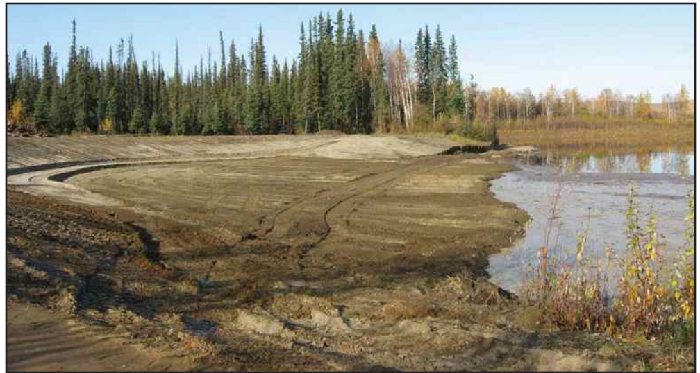
The steep sides of the former gravel pit are being contoured to create shallow littoral zones.
